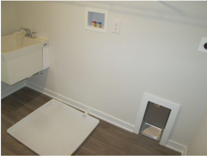
view of laundry room
