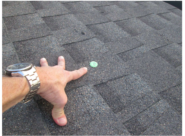
plastic tab and staple in shingle
