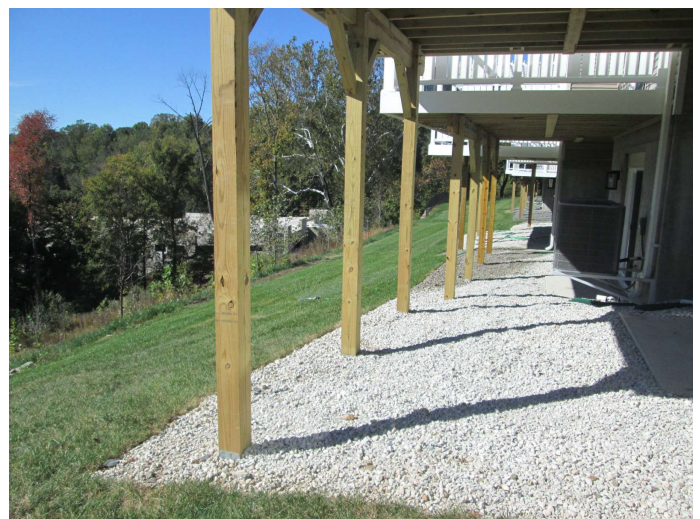
grades sloped away from house
