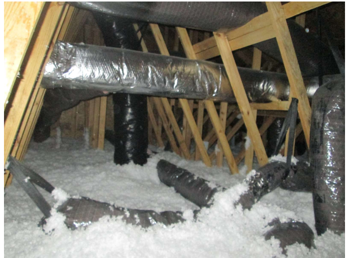
view of attic
