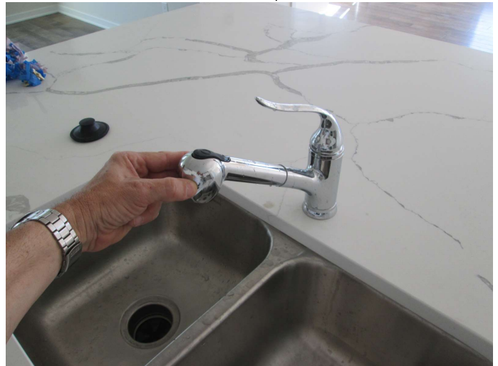
faucet not properly secured
