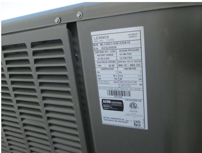
1 year old 4 ton AC condenser
