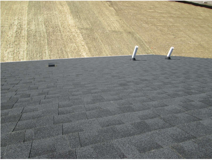
view of roof
