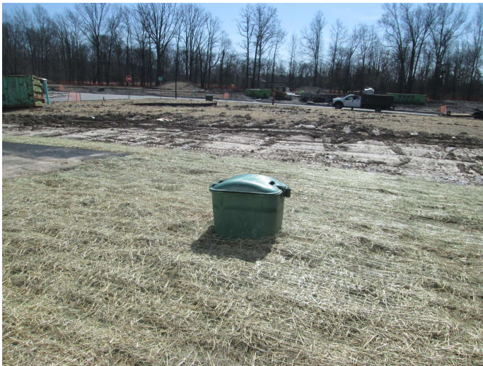
location of buried propane tank
