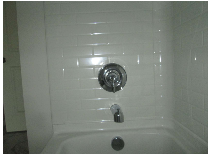
tub spout and faucet not aligned
