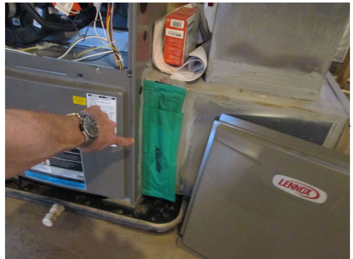
air filter cover not secure
