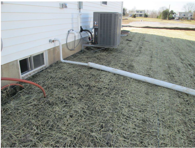
temporary extension of sump pump discharge pipe
