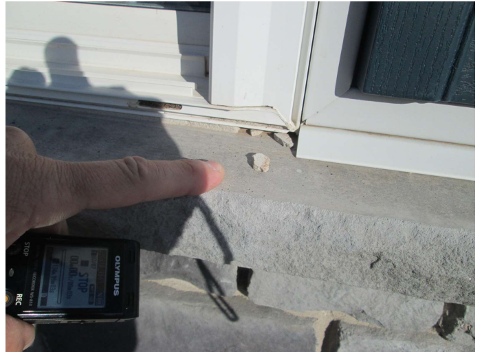
damaged pointing
