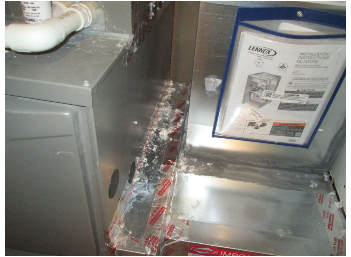
insulation from attic around zone #2 furnace (ceiling open to attic)
