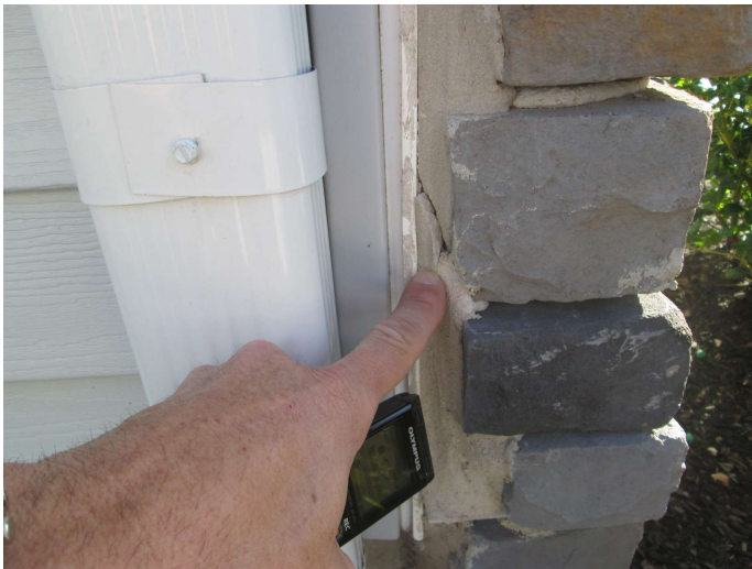
damaged pointing
