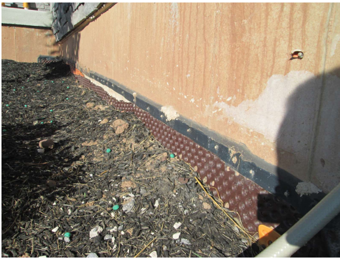
grades settled - foundation membrane exposed
