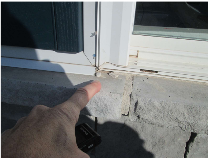
damaged pointing
