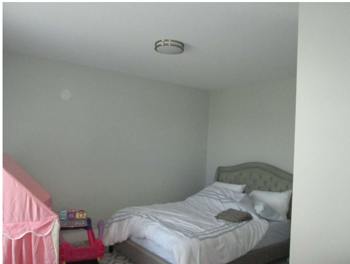
no smoke detector in basement bedroom
